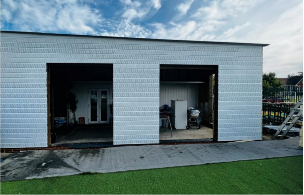
Side wall photo
